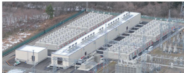
Storage battery system for the energy supply-demand control system
