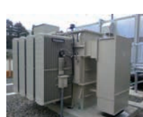
Canola oil-immersed transformer
