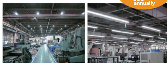
Replacing 400-watt mercury lamps with 200-watt LED models
