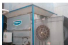
Well-closed cooling tower that takes water-saving needs into consideration
