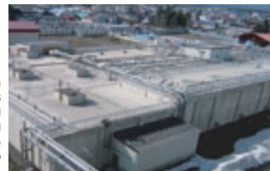
One of Japan's largest high-concentration organic wastewater treatment facilities (UASB methane fermentation, nitrification and denitrification, membrane-filtrated activated sludge, and biological desulfurization) delivered to a Hokkaido JA Shihoro potato starch plant
