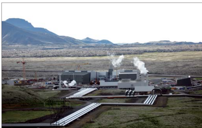
Hellisheidi power plant (in Iceland)
