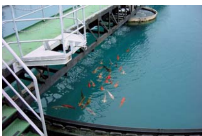
Wastewater treatment facility
