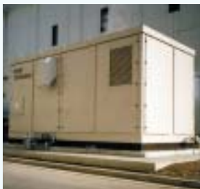
Sludge gas fuel cell power generation system
