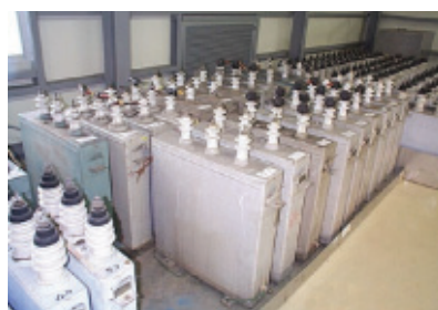
Storage of PCB-containing products on a tray
