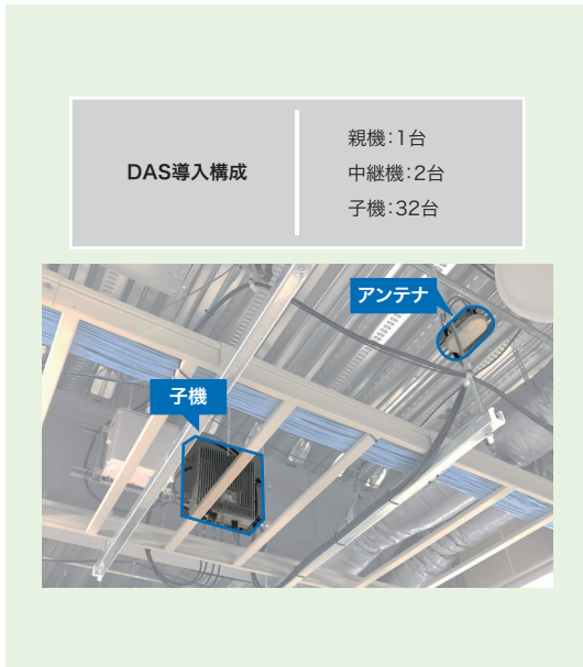
ローカル5G対応DASの設置例 Example of distributed antenna system (DAS) installation for local fifth-generation mobile communication system (5G) networks
