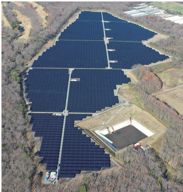
栃木県那須町の太陽光発電所 Solar power plant constructed in Nasu Town, Tochigi Prefecture
