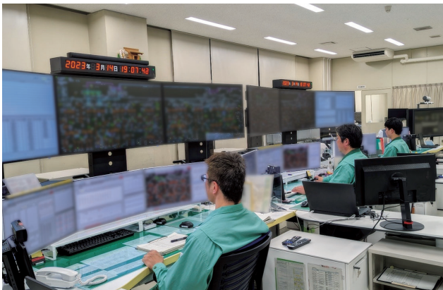
愛媛系制システム指令室 Control room at Ehime Grid Control Center of Shikoku Electric Power Transmission & Distribution Co., Inc.
