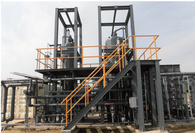
高速ろ過装置の実証試験設備 Pilot test equipment for high-rate sand filters with small footprint
