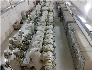
モサナ変電所の132 kV GIS 132 kV gas-insulated switchgears (GIS) installed at Al Mothana substation
