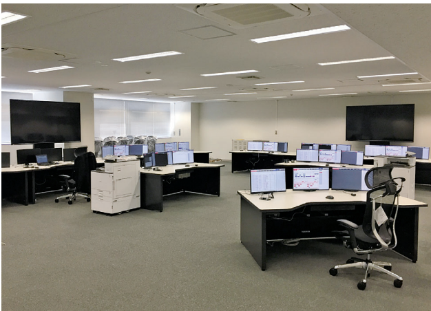
水力発電所集中監視制御装置 Central supervisory control and data acquisition (SCADA) system for hydroelectric power stations of TEPCO Renewable Power, Inc.
