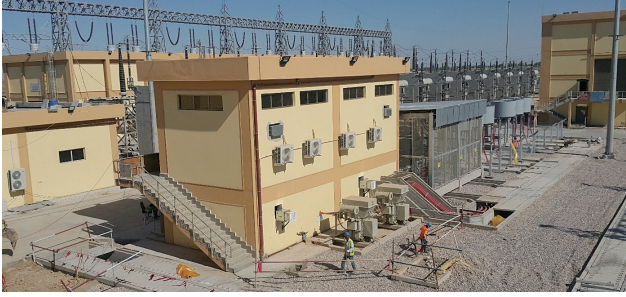
完成したイラクのモサナ400 kV変電所 Completed 400 kV substation located in Al Mothana, Iraq
