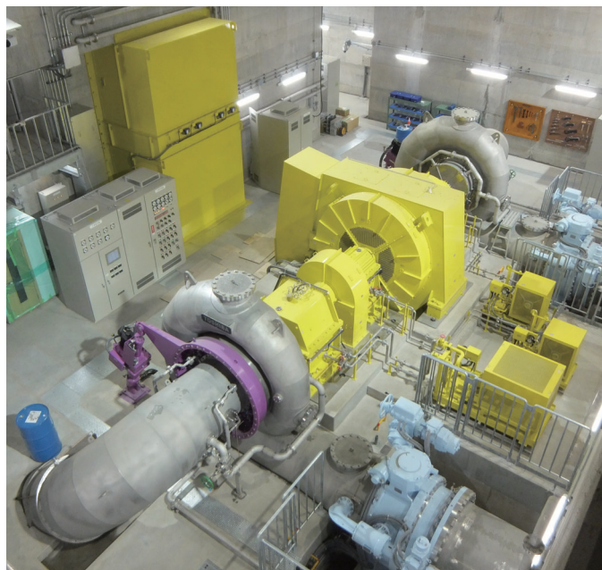
水車発電機 Hydraulic turbine generator for Yamba Hydroelectric Power Station
