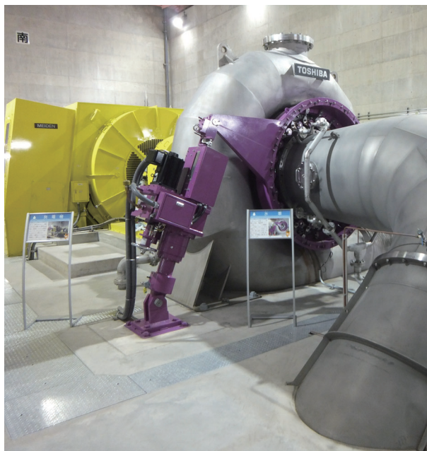
ハッ場発電所の水車 Hydraulic turbine for Yamba Hydroelectric Power Station of Gunma Prefecture
