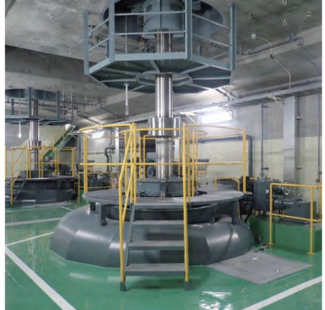
高千穂発電所の水車 Hydraulic turbine for Takachiho Hydroelectric Power Station of JNC Corporation
