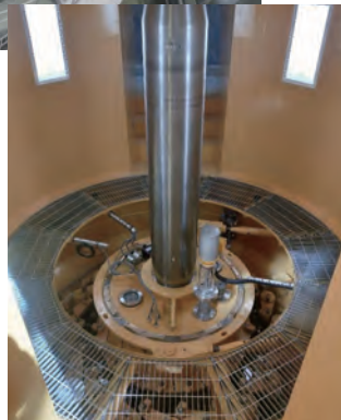
市房第二発電所の水車 Hydraulic turbine for Ichifusa No. 2 Hydroelectric Power Station
