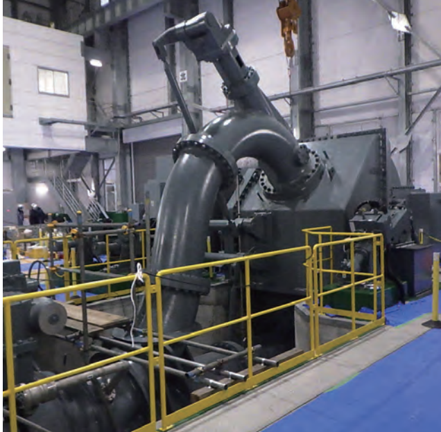
内大臣川発電所の水車 Hydraulic turbine for Naidaijigawa Hydroelectric Power Station of JNC Corporation
