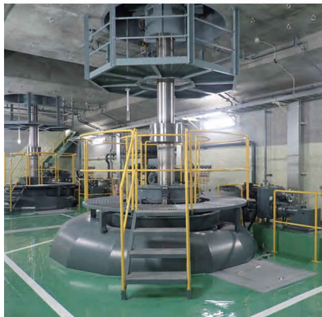
高千穂発電所の水車 Hydraulic turbine for Takachiho Hydroelectric Power Station of JNC Corporation
