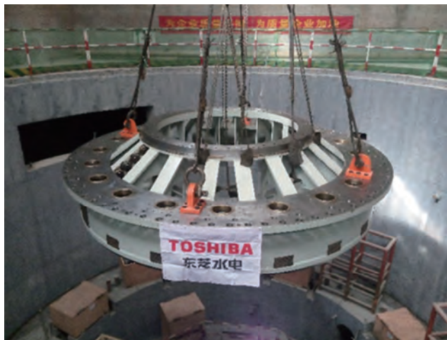
水車上カバーのつり込み Installation of turbine head cover at Jiangpinghe Hydropower Station, China
