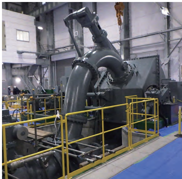
内大臣川発電所の水車 Hydraulic turbine for Naidaijingawa Hydroelectric Power Station of JNC Corporation
