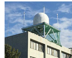
MP-PAWR radome installed in Saitama University
