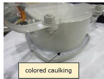
The area where the colored caulking compound is used
