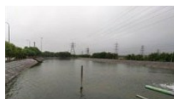
Pond for storing rainwater
