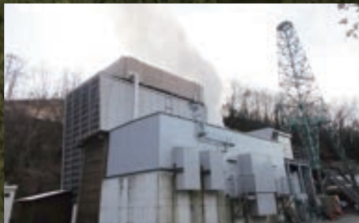
Waita Geothermal power plant
