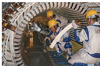
発電機補修 Electrical generator repairing
