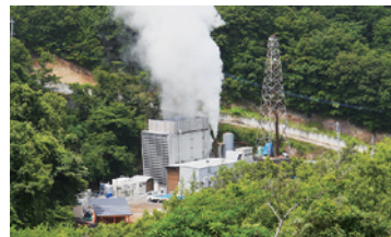
waita地熱発電所 (合同会社waita会様) Waita Geothermal Power Plant (Waita-kai LLC)
