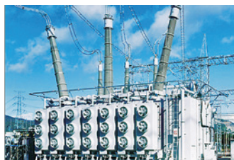
500kV-1000MVA 分解輸送型三相変圧器 (中部電力株式会社西部変電所) 500kV-1000MVA 3-Phase ASA (Advanced Site Assembly) Transformer (Seibu Substation of Chubu Electric Power Co., Inc.)
