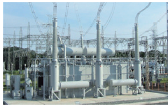
525kV-1000MVA 分解輸送型三相変圧器 525kV-1000MVA 3-Phase ASA (Advanced Site Assembly) Transformer
